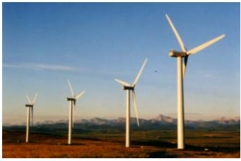
Plant capacity is 19.5 MW, generating 138 GWh/yr
